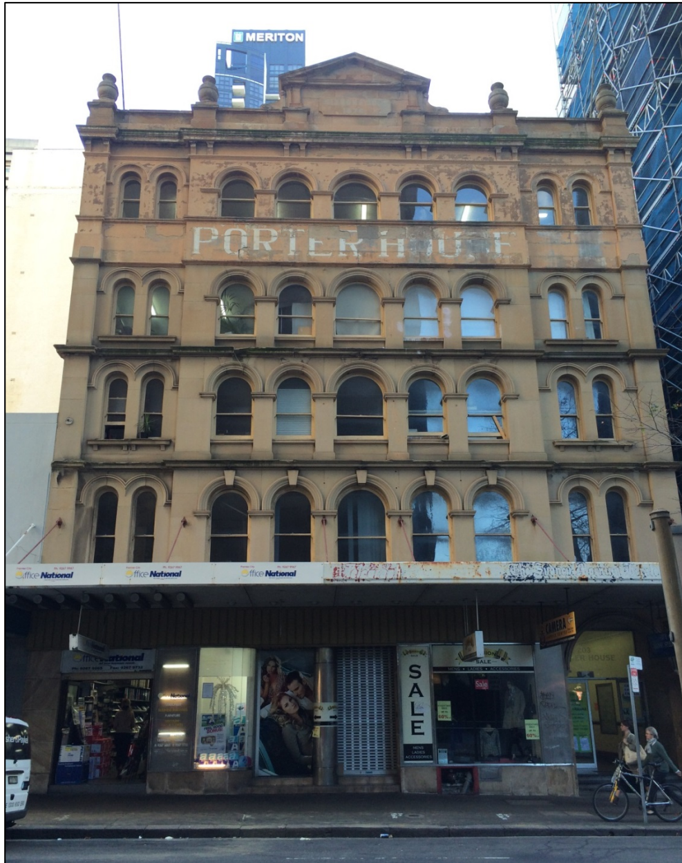
Figure 3: View of the existing 5-storey heritage building on the northern portion of the site, known as 'Porter House'
