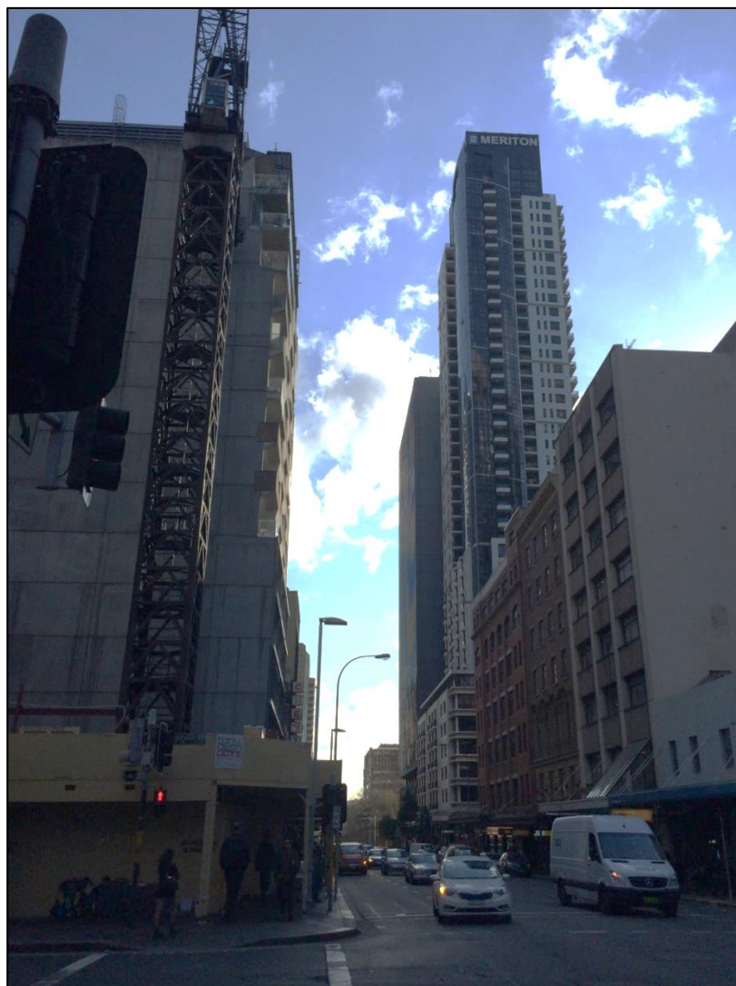
Figure 5: View of development surrounding the site looking west along Bathurst Street, including construction site (at 141-149 Bathurst Street) to the south of the site
